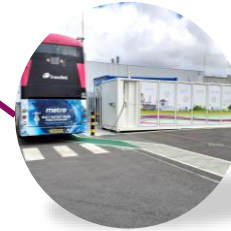
Milewater Service Centre Hydrogen Refuelling Station
